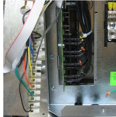
8- Move the protector to the left side of the boiler in order to access the power board
