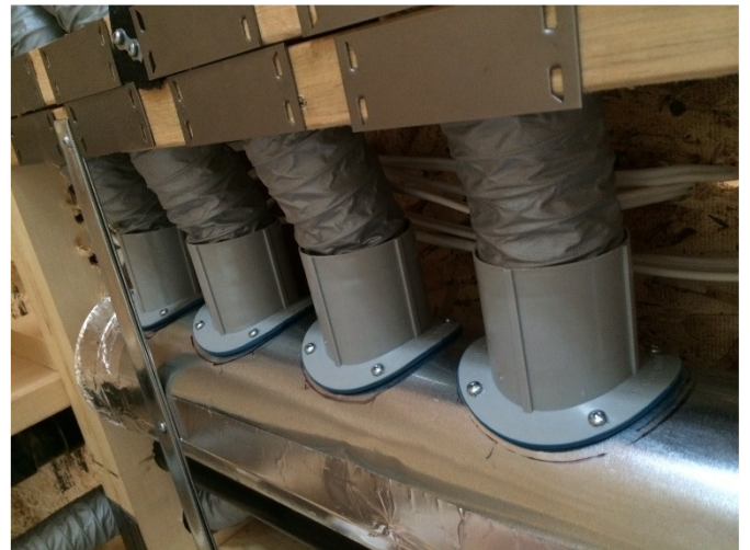
Figure 21: Screw the saddle on the trunk
