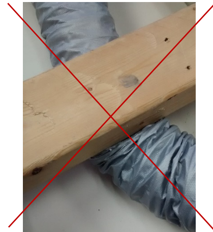
Figure 9: Do not crush the flex duct
