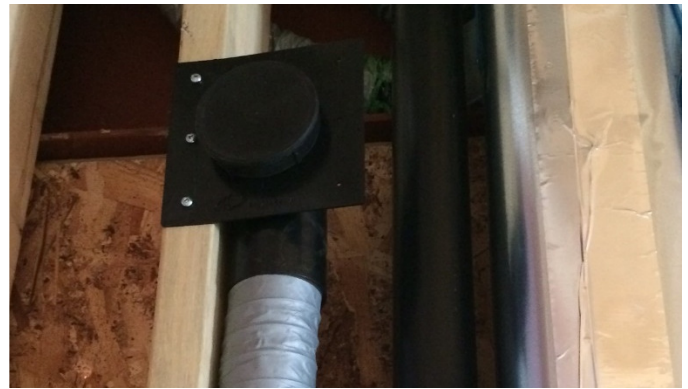
Figure 22: Attach the collar on the wall stud
