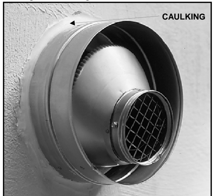
Figure 6 : Caulking around the stabiliser shroud
